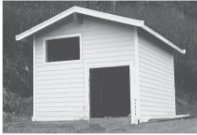
The littlest house in Port Ludlow is home to the new South Bay pumping station.
