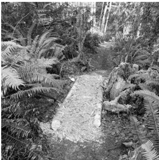
Corduroy pathway built on Creek View Loop to relieve muddy section
